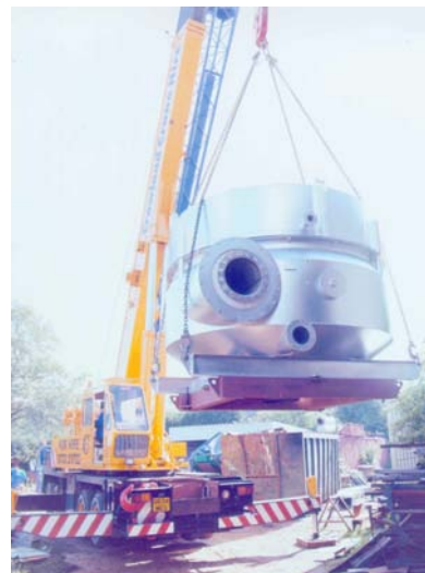
A Catalyst Processor is hoisted into position
