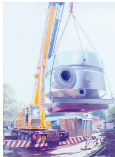
A Catalyst Processor is hoisted into position
