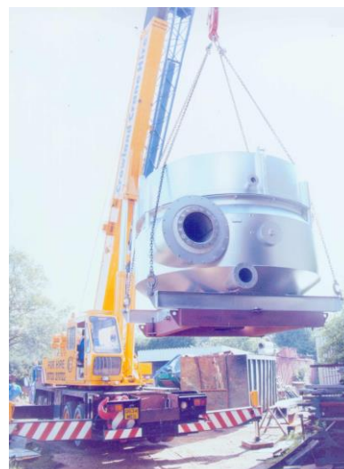
A Catalyst Processor is hoisted into position
