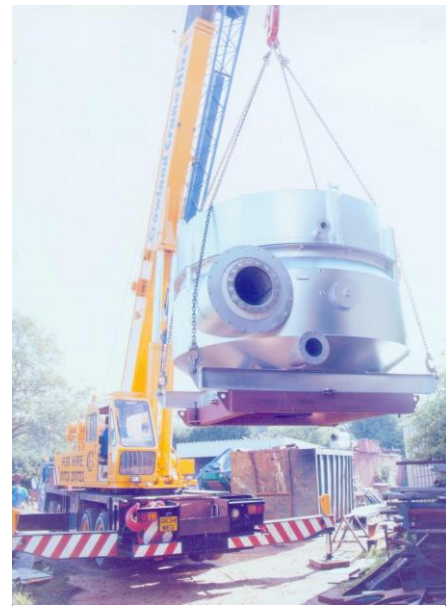
A Catalyst Processor is hoisted into position
