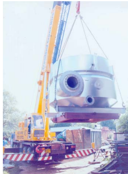
A Catalyst Processor is hoisted into position
