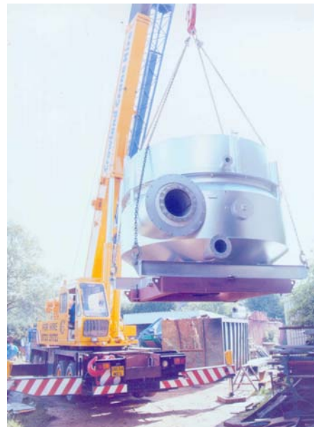
A Catalyst Processor is hoisted into position
