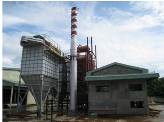
A 2MWe TORBED Rice Husk Combustor under construction in Cambodia
