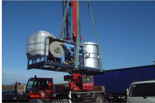
Figure 1: TORBED T1000 Module being installed
