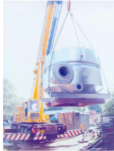
A Catalyst Processor is hoisted into position
