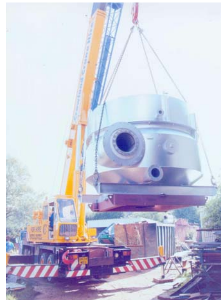
A Catalyst Processor is hoisted into position
